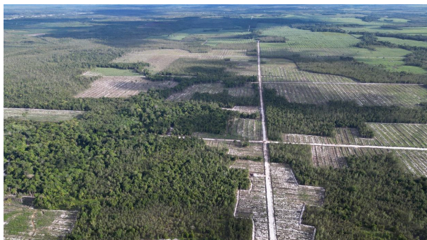
Road and plantation development causing fragmentation of natural forest in PT IFP's concession
